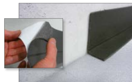
(4) Cover the junction between the underlay and the wall with the peripheral strip Lfoam
