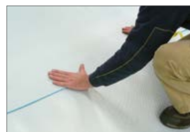
(3) Stick correctly the two layers together
